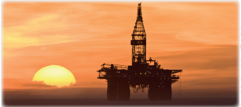
Drilling data analysis on-site
